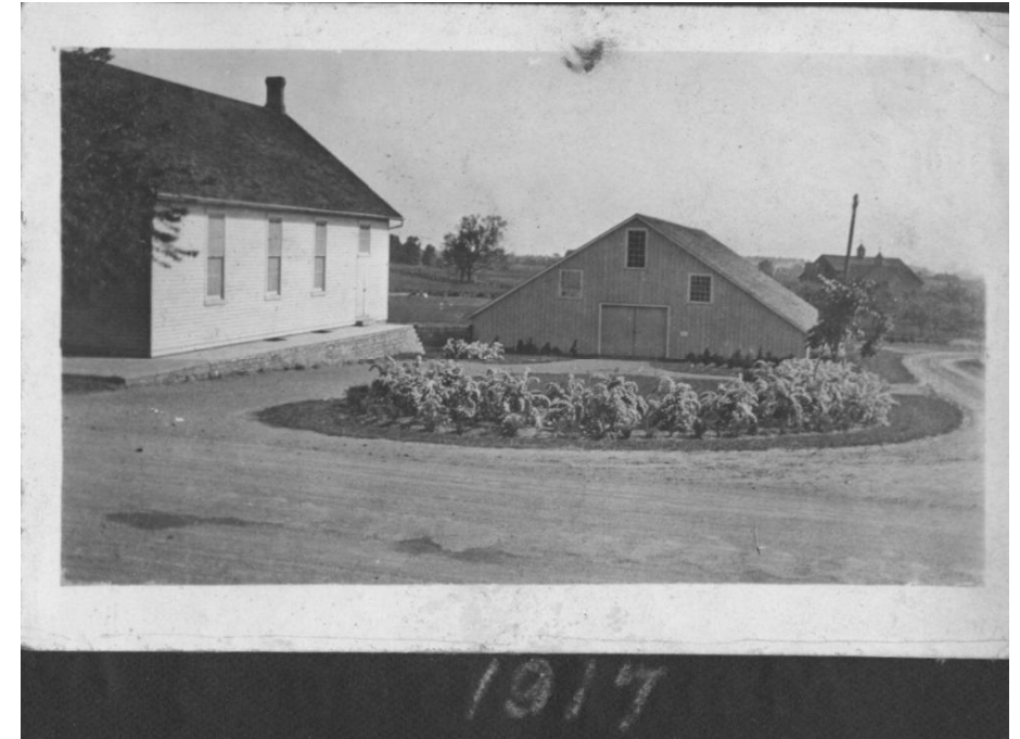
Vineland Mennonite Church – Drive Shed (used to store buggies and cars of church goers)
