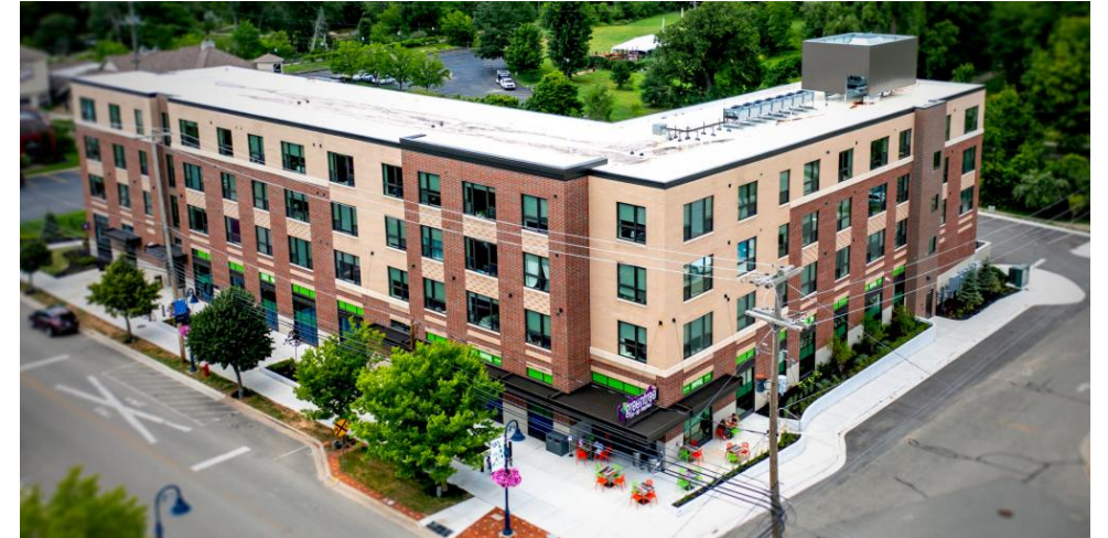
Broadway Lofts (Mt. Pleasant, MI) – Ground Floor Grocery Store, Parking at Rear
