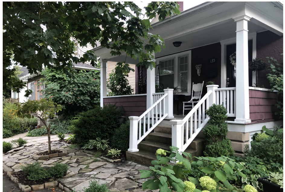
Figure 11: Generously sized covered porch provides functional outdoor living room and activates streetscape
