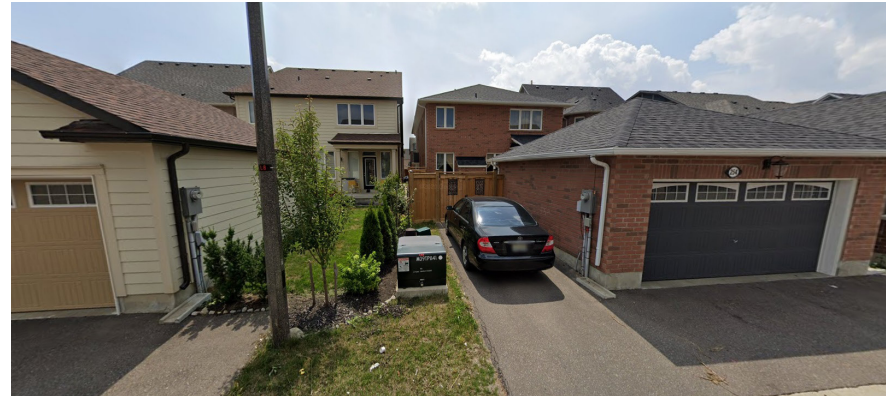
Figure 19: Typical rear lane garages
