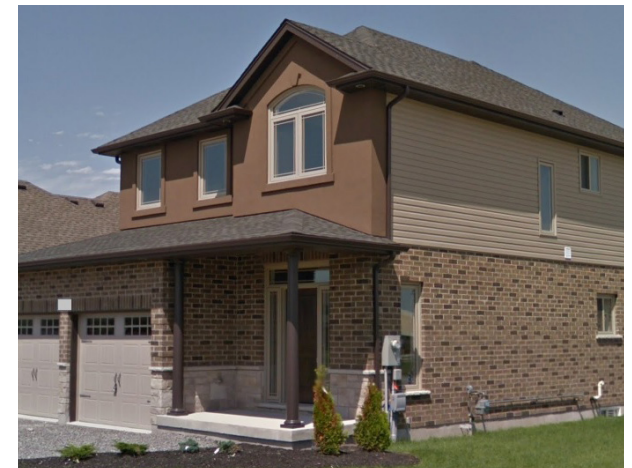
Figure 6 Excessive variety and imbalanced cladding arrangement
