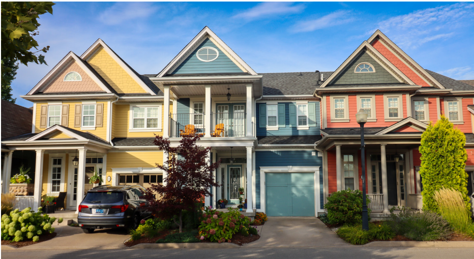
Figure 12: Proper window & door alignment paired with functional covered balconies
