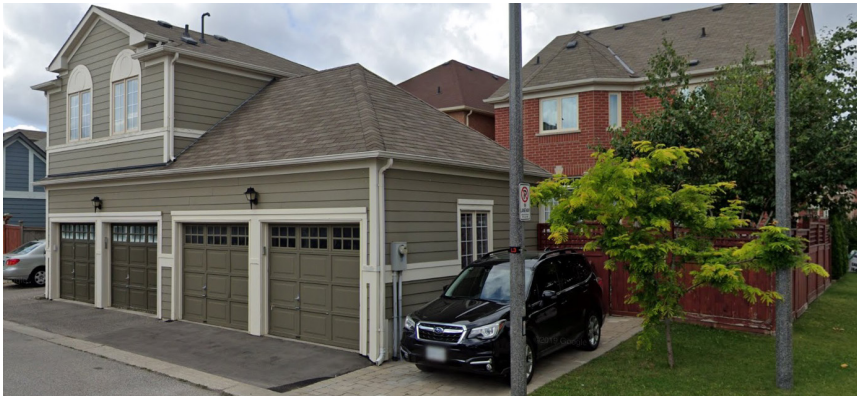
Figure 18: Pre-finish sided garages serving brick houses
