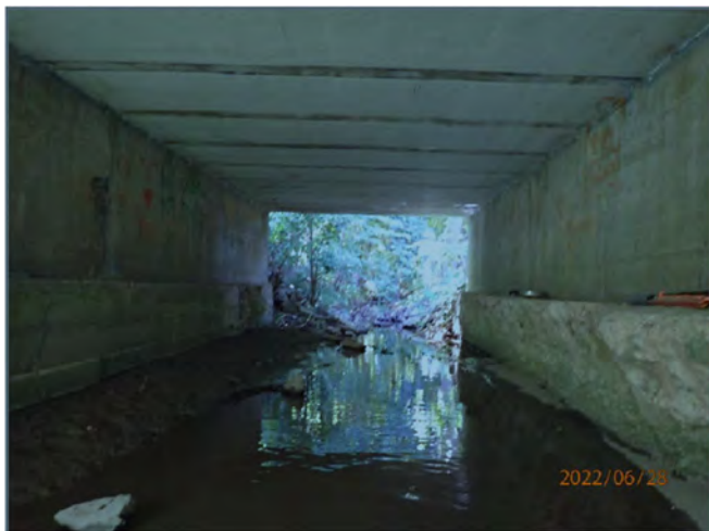
Existing Box Culvert
