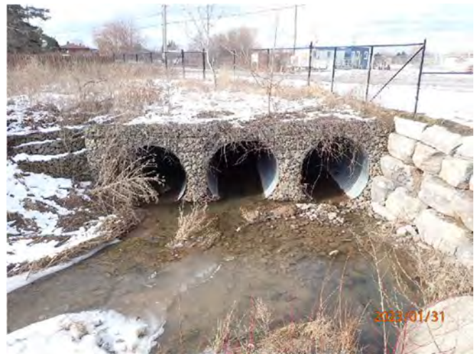
Triple CSP Culvert
